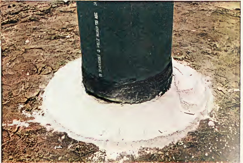
A 18: TOP LAYER OF BENTONITE APPLIED
